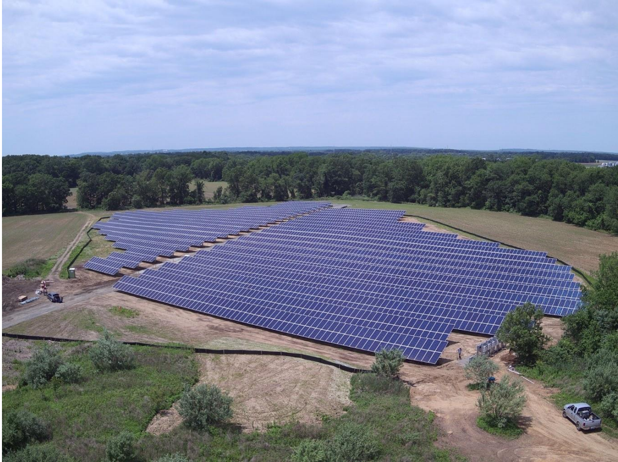
Fig. 22 – 1.7 Mega Watt Solar Field
