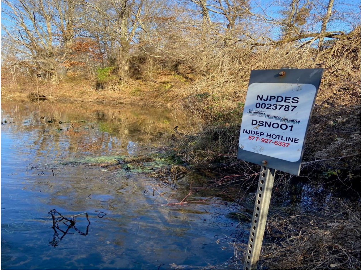
Fig. 23 – East Windsor MUA NJPDES Permit – Outfall Pipe
